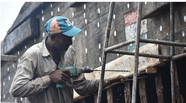
Fig. 1 Replacement of wooden plank in progress
