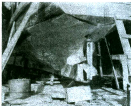
Fig. 1 — Final stages of sheathing
