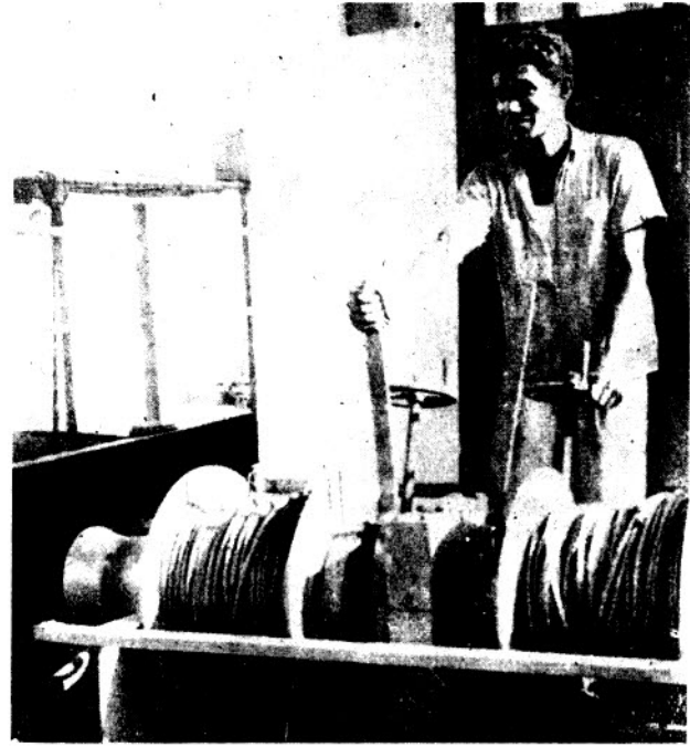
A trawl winch of the Institute's design in operation
