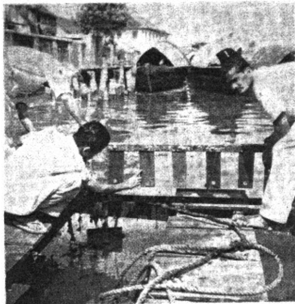
Wooden test panel is being examined for the effect of Marine Borers and Foulers
