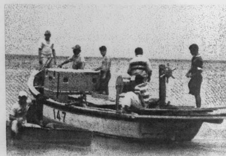
Installing insulated FRP fish hold in the boat
