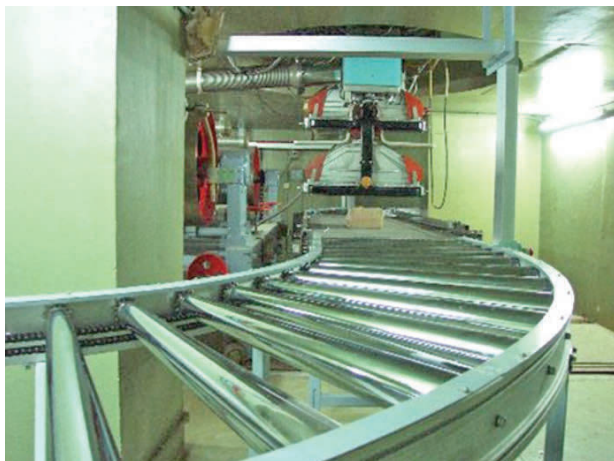
Fig. 1. Electron Beam Processing Section of IRAD, BARC
