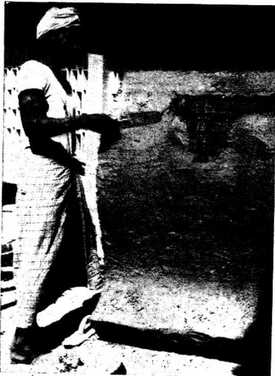
Fig. 6 The reinforcement is filled and covered with cement and sand mortar.
