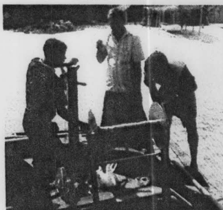
Modification works in progress
